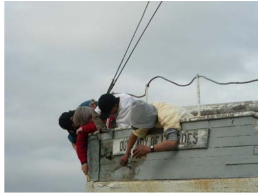
Refurbishing the Lady of Lourdes
